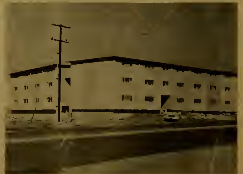
New McAfee Apartments NEAR completion.
